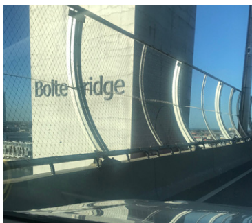
Bolte Bridge Safety Barriers
