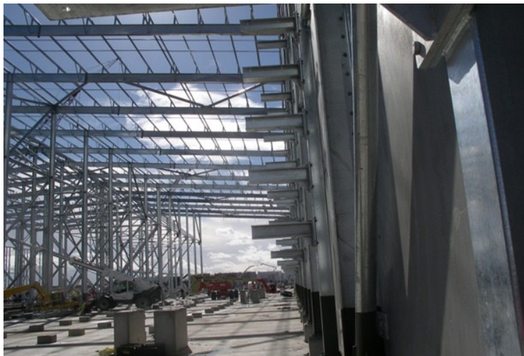
Desalination plant, Sydney during construction – the lower section of the uprights are painted to protect the surface from salt splash
