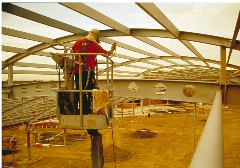
Primer being applied over galvanizing to EG Whitlam Pool frame structure in preparation for decorative coat
