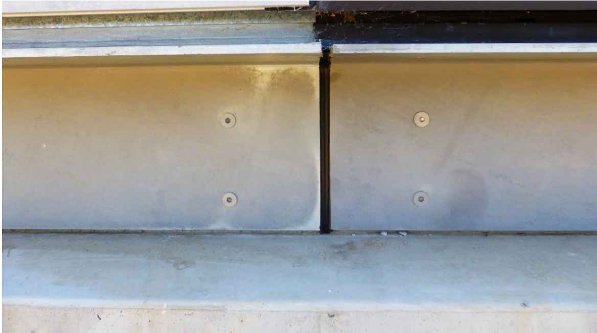
Figure 1: A dull grey appearance on some steel beams due to the chemical composition of the steel.
