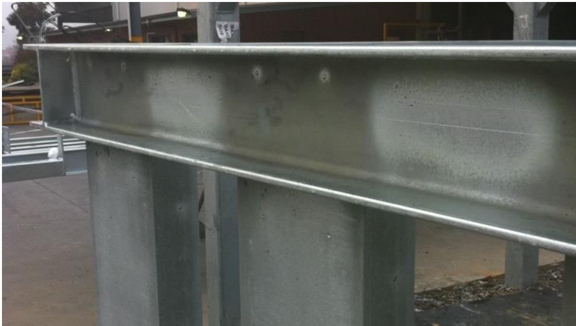
Figure 3: A dark grey coating is seen where steel is held at a higher temperature for longer and alloy layers can continue to form. More examples of both shiny and dull regions on the same article can be found in Differing Appearance .
