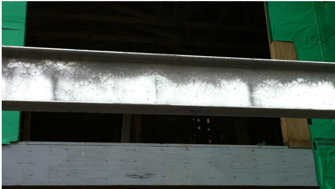
Figure 4: The darker section of this beam has likely spent more time over the galvanizing bath while the zinc drains off. The mottled appearance is indicative of the alloy layers growing to the surface in some places.
