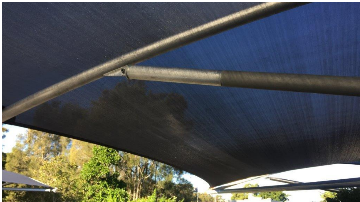
Figure 11: A circular hollow section comprising of steel with different compositions holding up a shade cloth. The colour different is purely aesthetic and has no influence on the corrosion resistance of the part.
