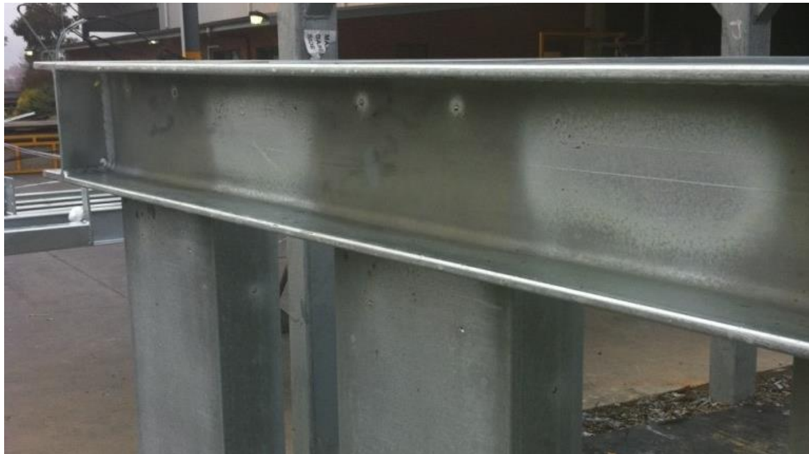
Figure 3: The thick steel behind the beam has caused slower cooling of the web in places, resulting in a duller coating.
