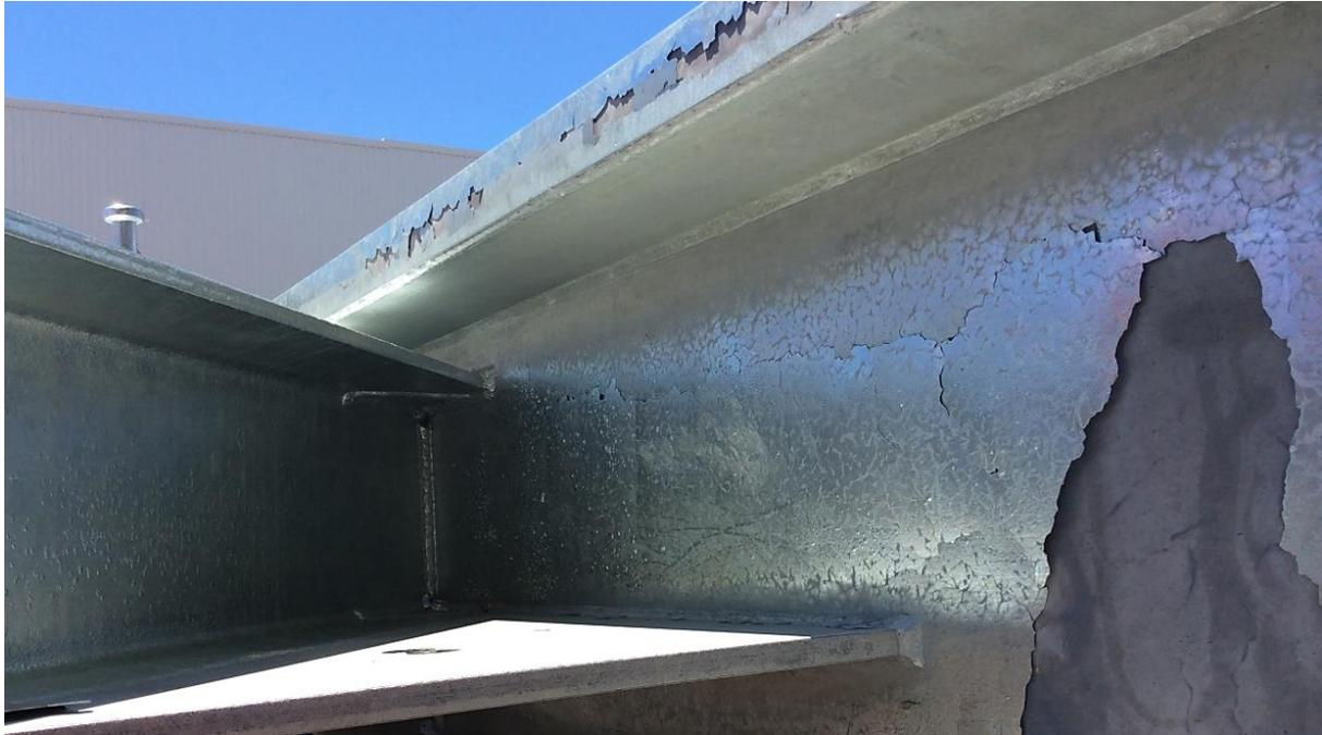
**Figure 1:** The galvanized coating is flaking off on multiple places of the article. Depending on the size of the bare spots and end use it may need to be regalvanized.
